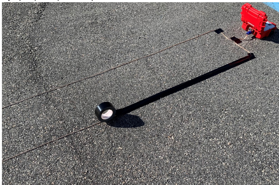
Fig 6. Taping the loop wires down with gaffers tape. A white finishers line can be placed in the middle of the tram lines.
